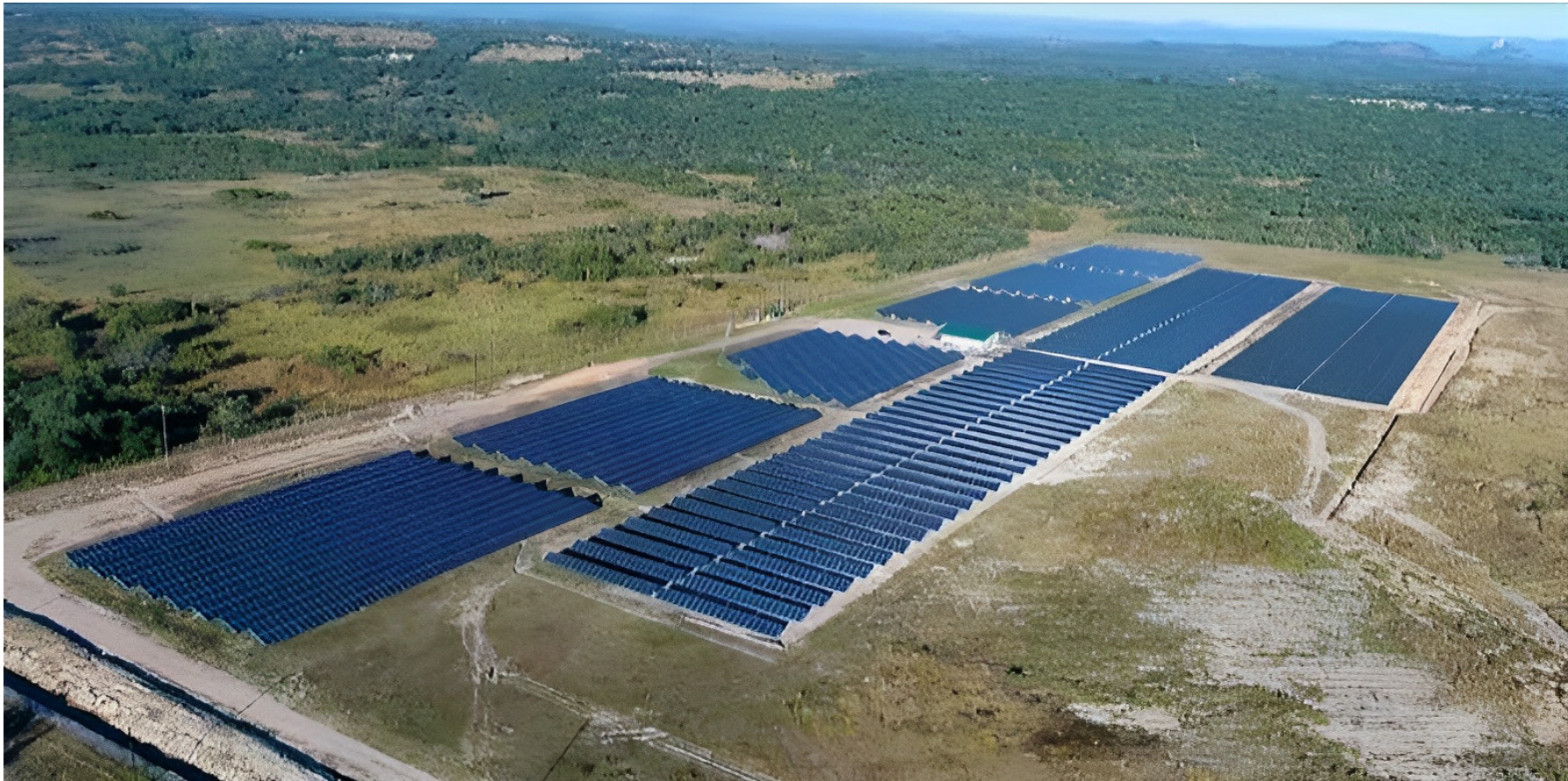
Figure 4: Zimbabwe's first purpose-built grid tied solar PV station with 2.5 MW installed capacity. Image courtesy of NRE Zimbabwe
